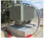
Special extinguishing frames assembled on prefabricated concrete retention tanks or small pit etc....
